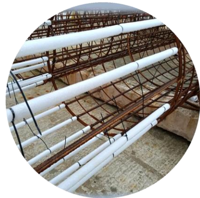
Rebar protection application
