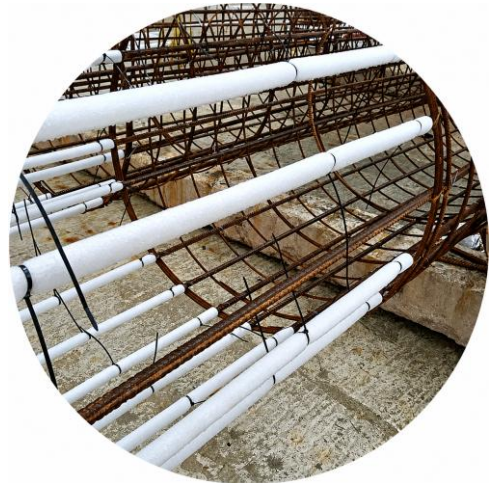
REBAR PROTECTION IN USE
